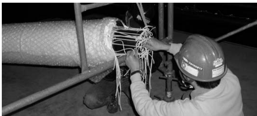
Figure 10. Rigger attaching tie cords to tube end on elevated screen
