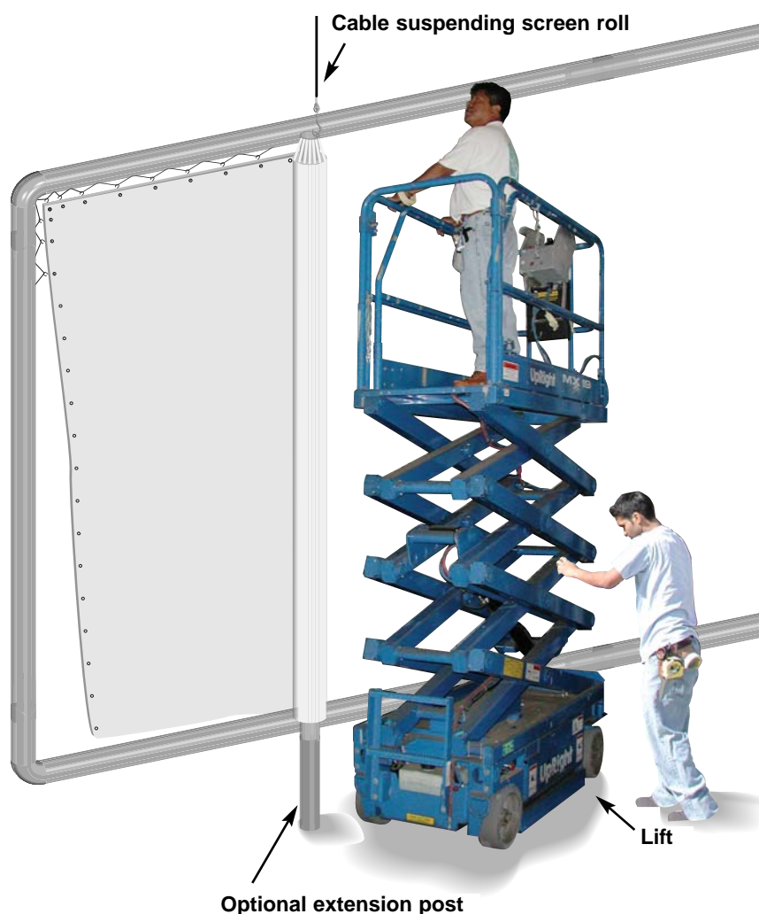
Figure 13. Beginning to attach screen to frame
