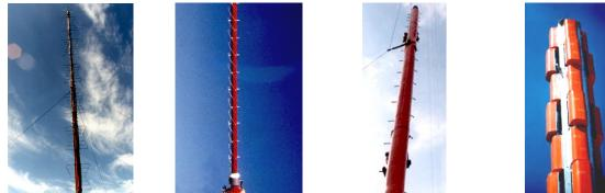
Fig 11 – High gain antennas used by TV transmitters
