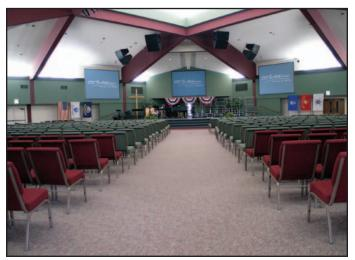
A point-and-shoot system was the appropriate choice at Mountview Church in Olympia, WA, designed and installed by CCI Systems. Shown here are PD5212 loudspeakers (/64 for long-throw and /95 for short-throw) from JBL's Precision Directivity Series.
